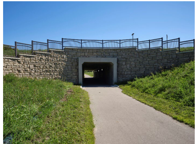
FIGURE 3: PEDESTRIAN TUNNEL UNDER CSAH 101
