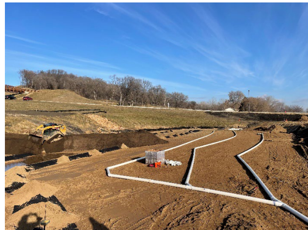
FIGURE 4: DRAIN TILE CONSTRUCTION FOR STORMWATER BMP
