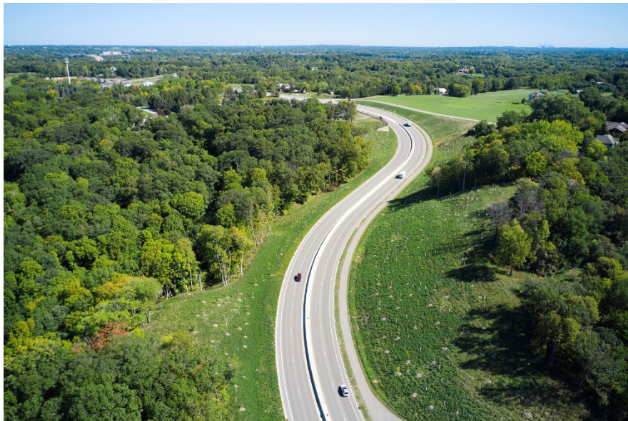
FIGURE 2: NEWLY CONSTRUCTED CSAH 101
