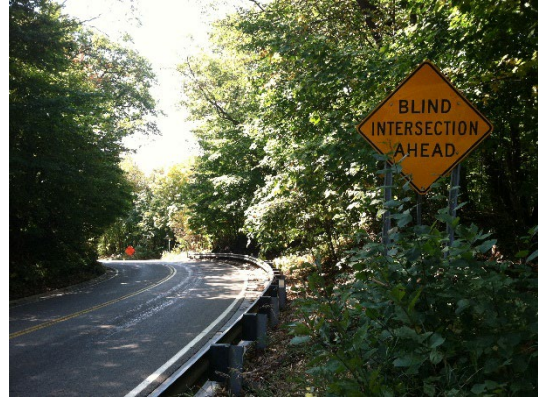
FIGURE 1: EXISTING CONDITIONS SHOWING TIGHT CURVES AND STEEP GRADE
