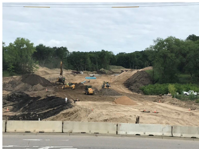
FIGURE 5: EARTHWORK OPERATION TO REMOVE 430,000 CY OF MATERIAL
