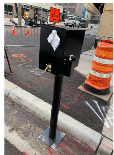
Example of a hand washing station used during Hennepin Avenue Downtown construction.
