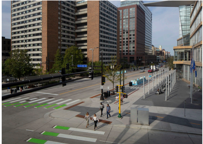
The design of Hennepin Avenue Downtown included innovative design treatments including tactile guide strips, railings, and colored pavement at the transit stations.
